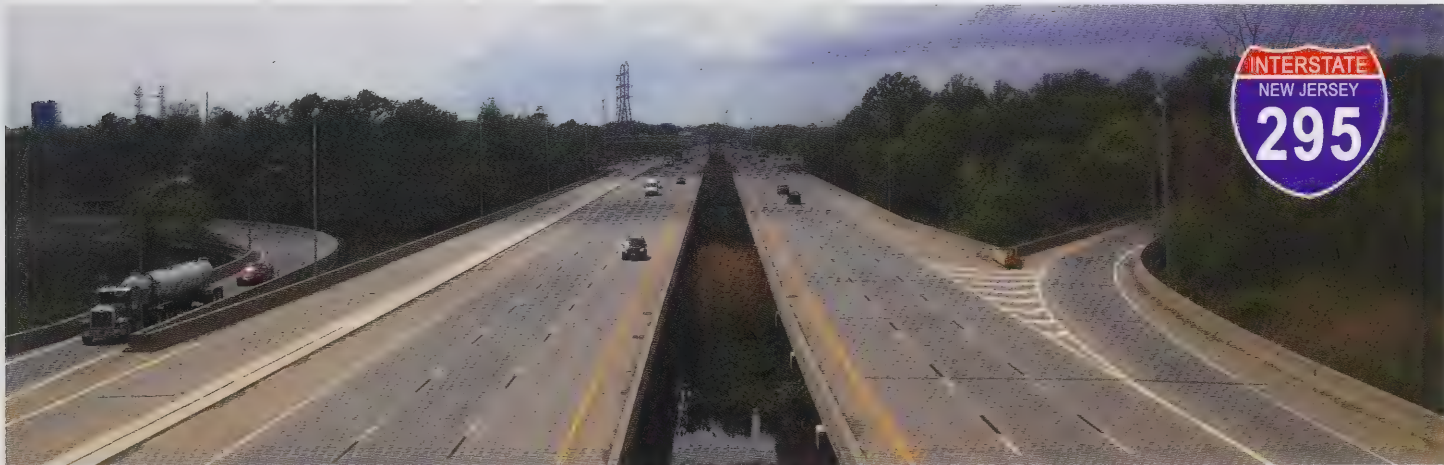
NJDOT opened the 5.5 mile section of I-295 connecting to I-195, as part of the Trenton Complex. (1987)
